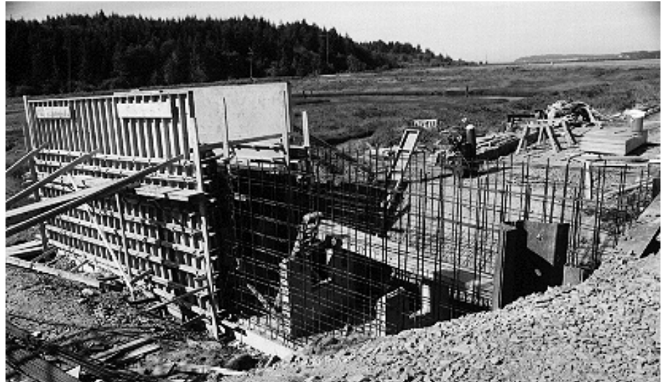
The new fish ladder under construction at the Lewis Unit in August was a forest of rebar flanked by plywood forms. The ladders were estimated to take about four months to put in.
